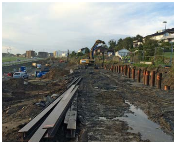
Montering bjelkestengsel.
