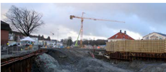
Utgraving for betongkulvert Madlaveien i St. Svithun-parken. Her skal vi 15 meter ned.
