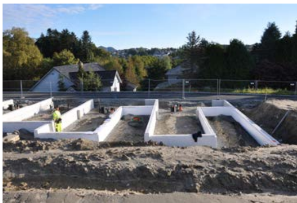
Ringmurer for rekkehus Sandsgård
