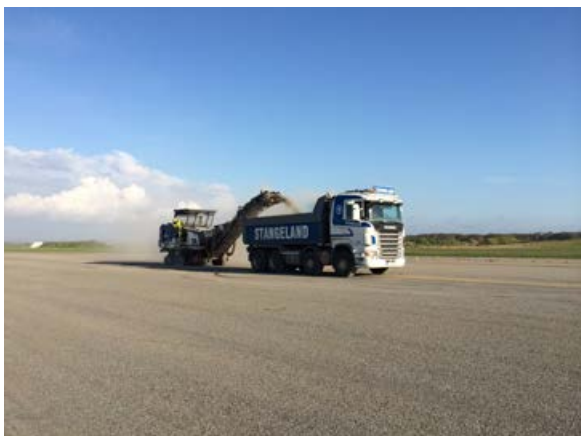
Reasfaltering rullebaner – fresing 2
